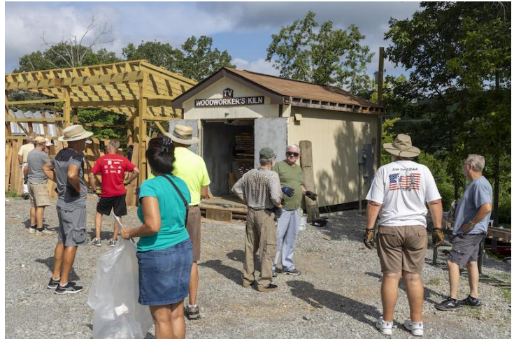
New Kiln under construction & Old Kiln
